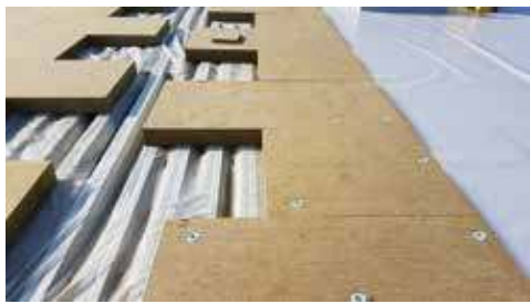
Metal deck with FIBRANgeo BP 70 boards and waterproofing membrane on top.
